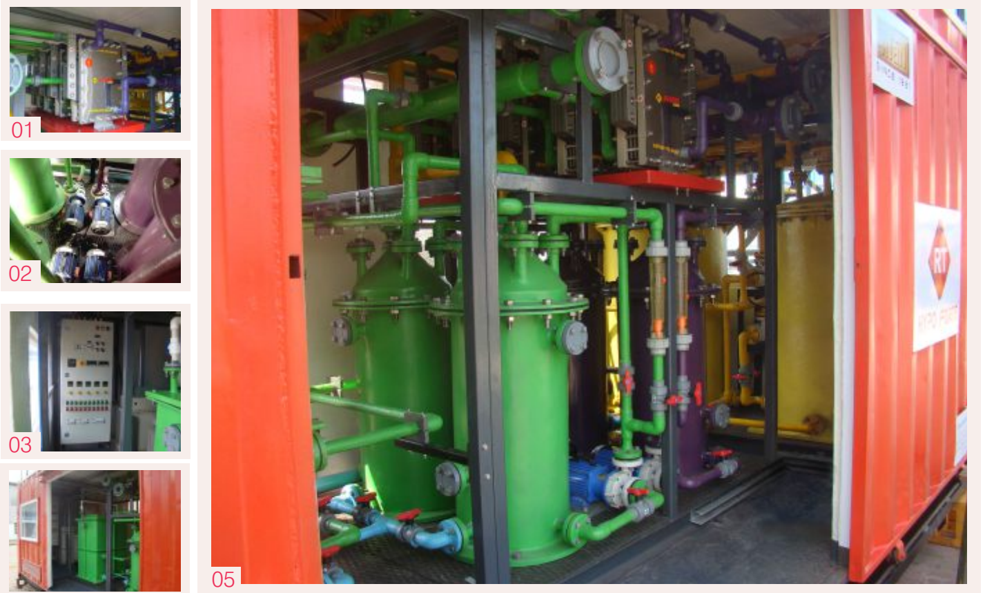
01. MEMBRANE ELECTROLYZER 02. ANOLYTE / CATHOLYTE 03. CONTROL PANEL 04. BRINE SECTION 05. RT HYPOFORTE SYSTEM
